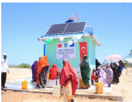
Solar-powered water point.
